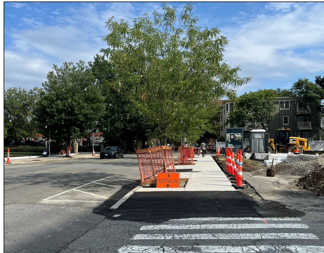
Broadway at MBTA Busway, September 2026
