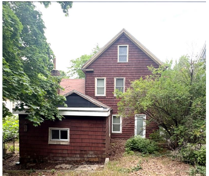
Above: Rear elevation of 83 Wallace St
