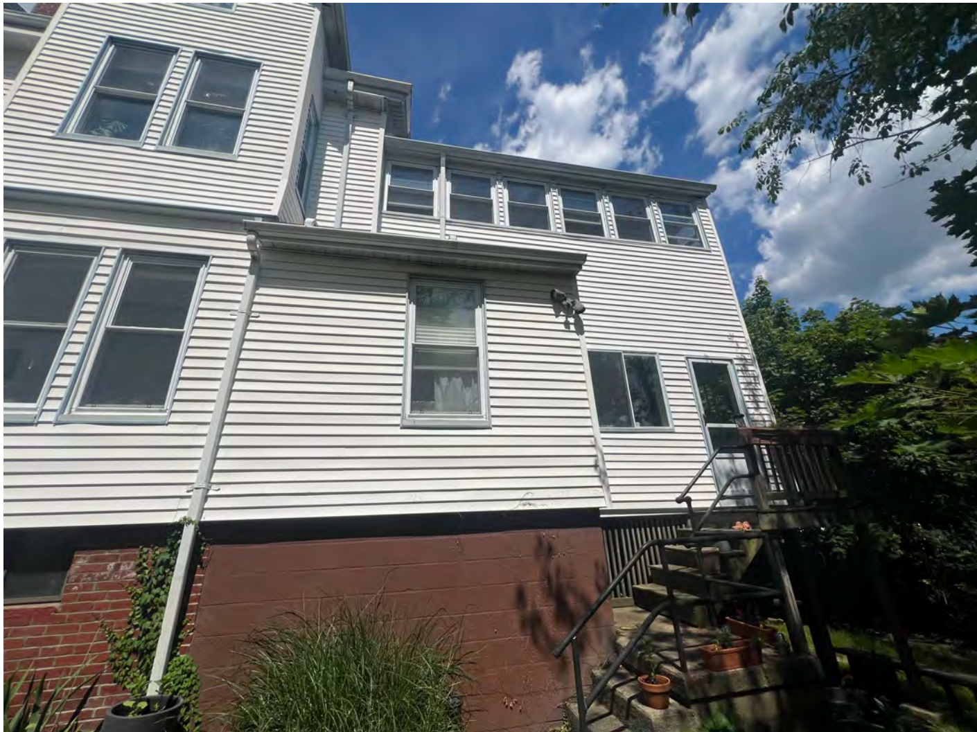
EXISTING VIEW OF AREA FOR PROPOSED PORCH FROM RIGHT SIDE YARD
