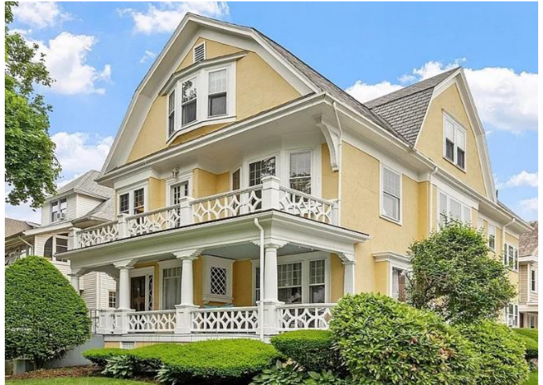
Front Elevation of 52 Powder House Blvd.
