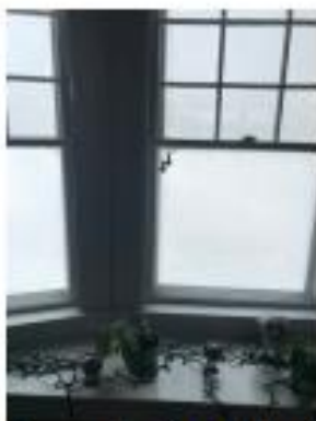
Example of window frosted over in winter given lack of proper insulation
