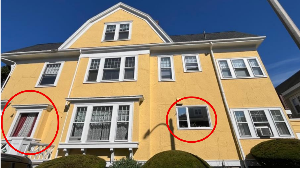
Above: Right side of 52 Powder House with original windows proposed to be replaced circled
