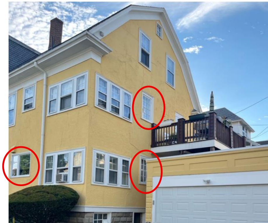
Above: Rear of 52 Powder House with original windows proposed to be replaced circled
