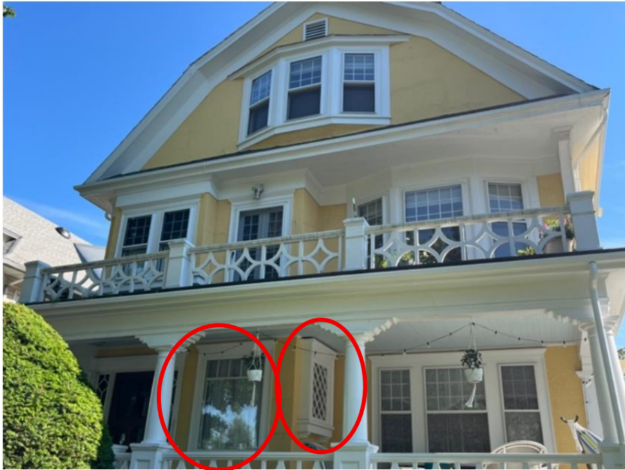
Above: Front of 52 Powder House with original windows proposed to be replaced circled
