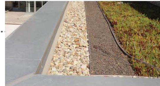
Extensive Sedum Green Roof with Crushed Stone Ballast
