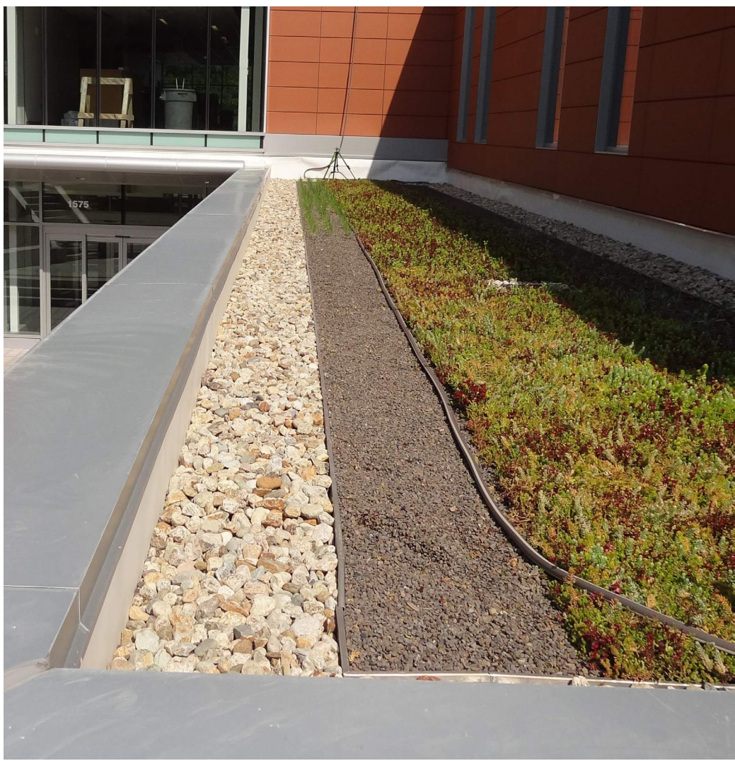
Extensive Sedum Green Roof with Crushed Stone Ballast
