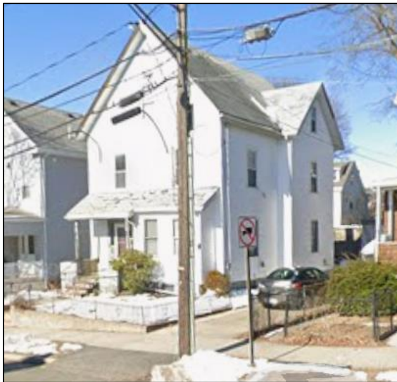
Above: Right façade in 2022, prior to construction
