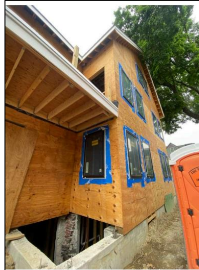
Above: current front facade
