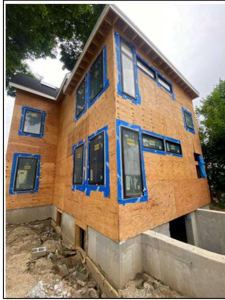
Above: current rear facade
