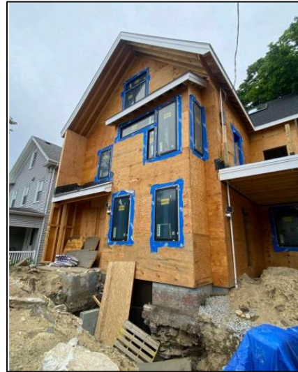
Above: current front facade
