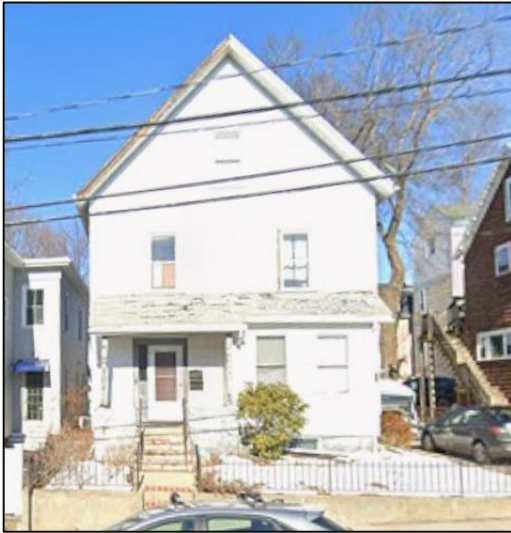
Above: front façade in 2022, prior to construction
