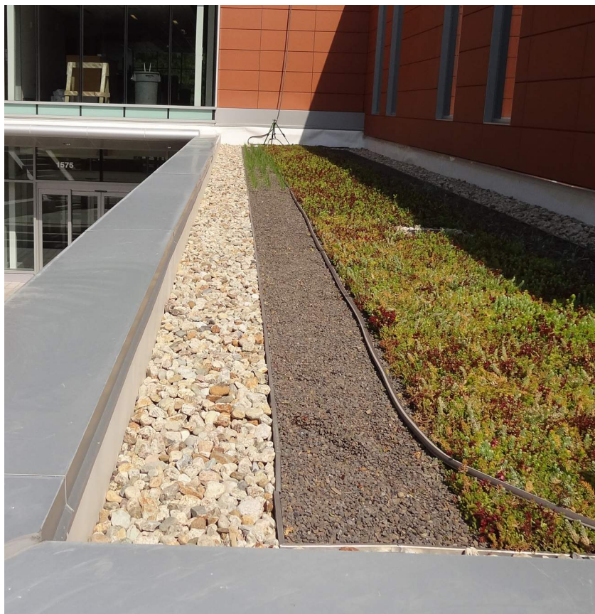
Crushed Stone Ballast and Sedum Green Roof
