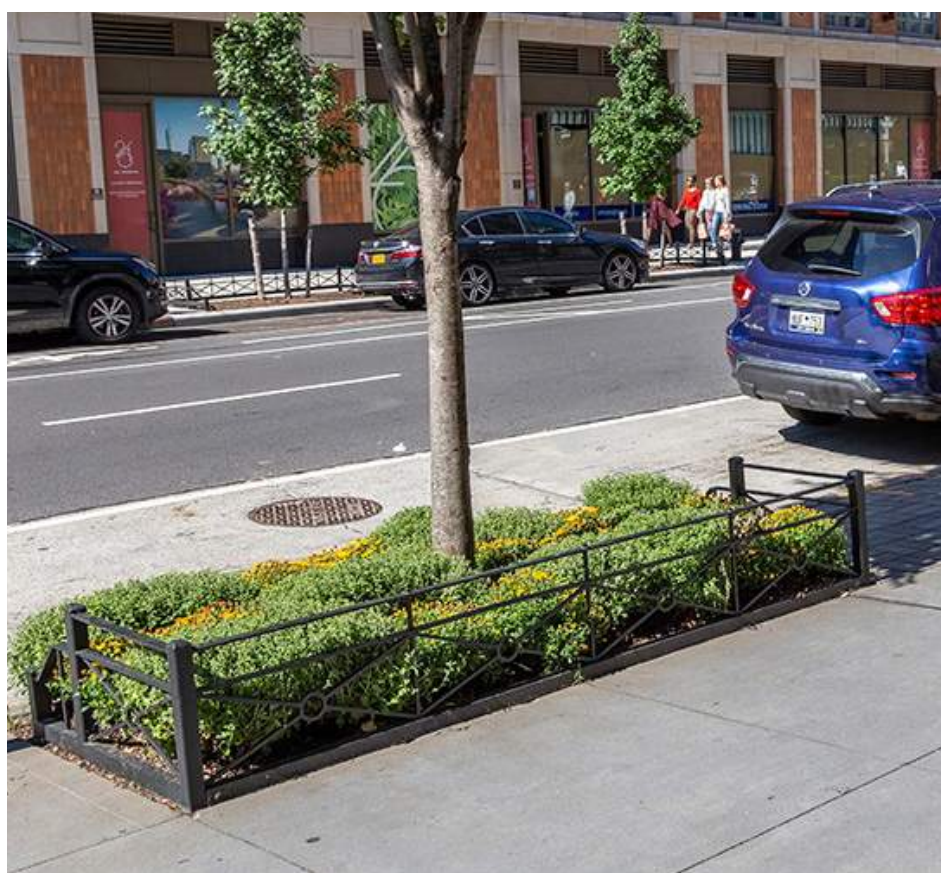
18" Ht. Tree Guard at Street Trees Along White Street
