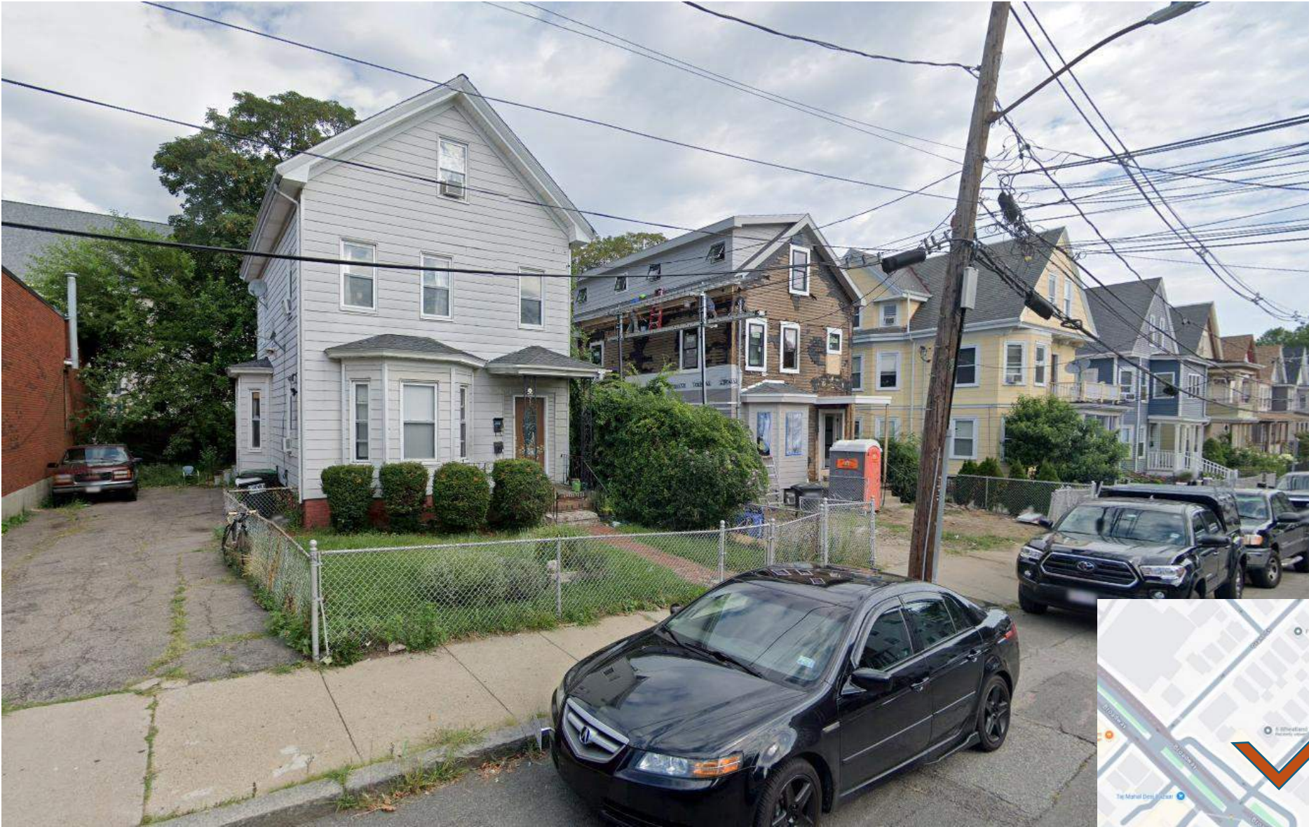
6 Wheatland Street, Somerville, MA Existing Conditions
