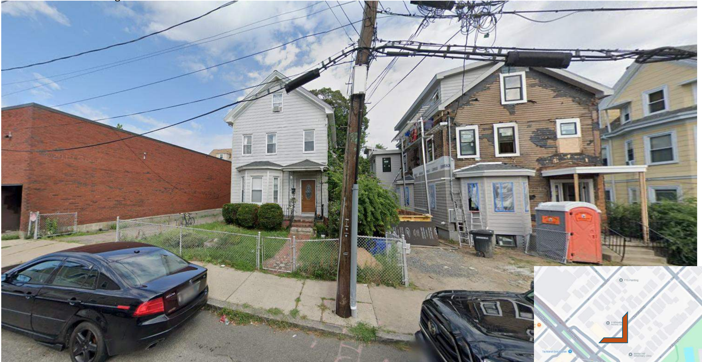
6 Wheatland Street, Somerville, MA Existing Conditions
