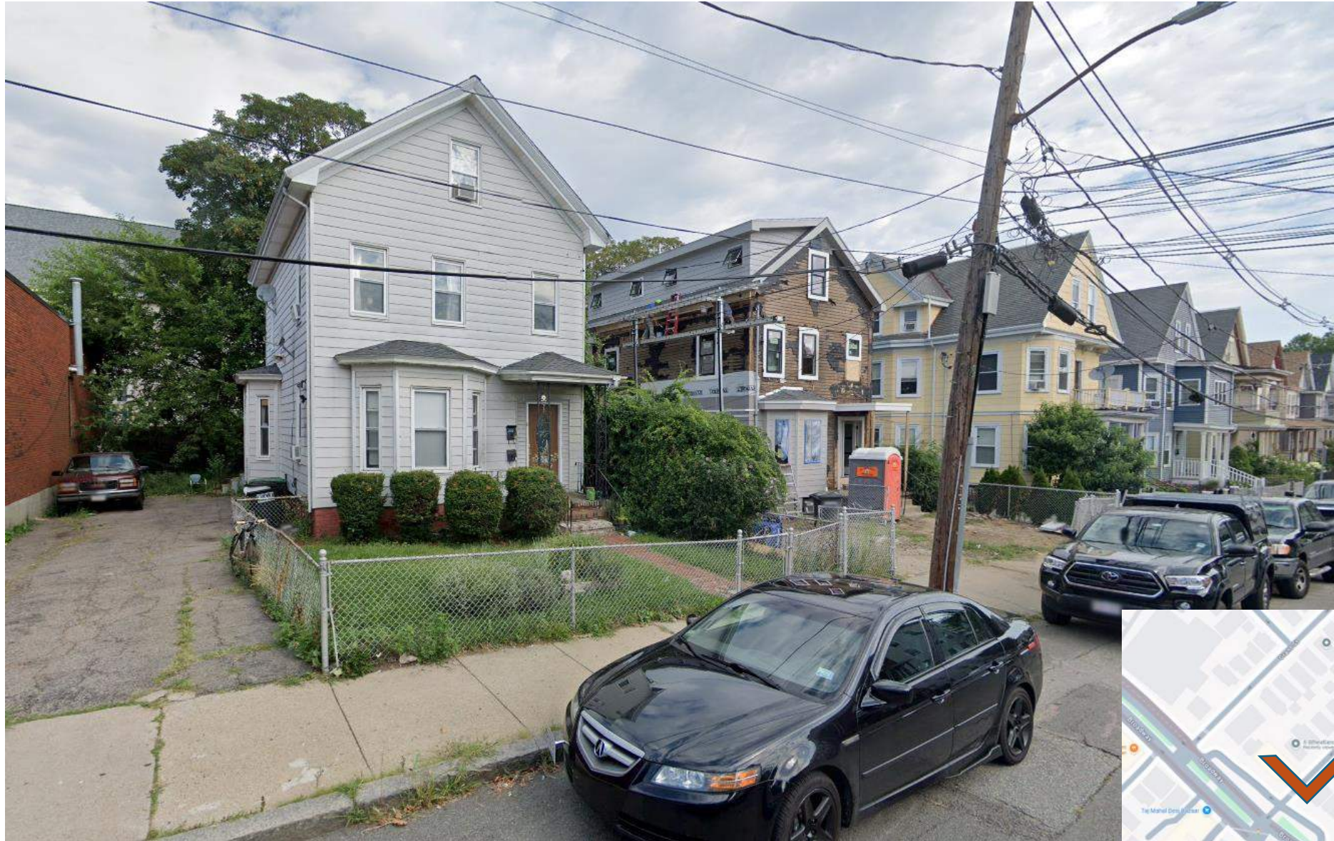
6 Wheatland Street, Somerville, MA Existing Conditions
