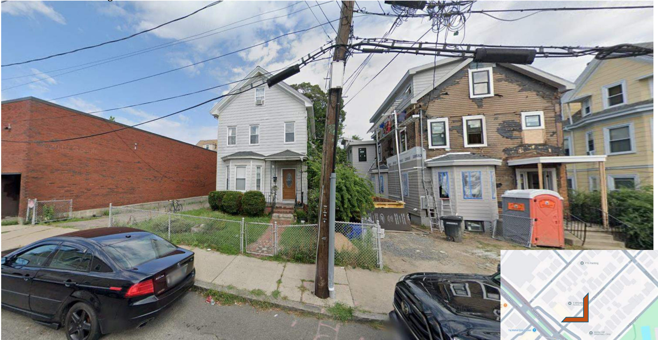
6 Wheatland Street, Somerville, MA Existing Conditions
