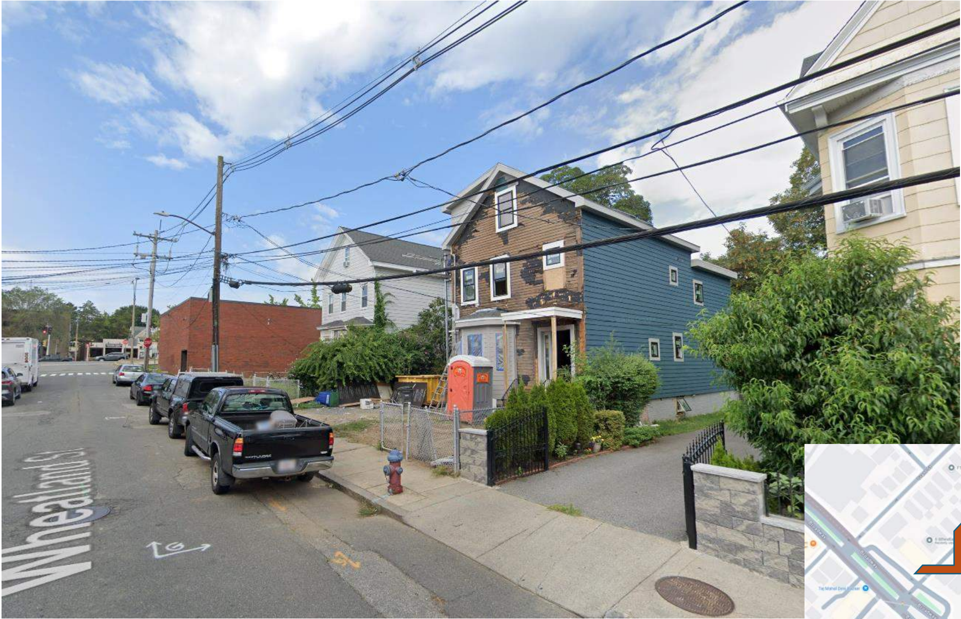
6 Wheatland Street, Somerville, MA Existing Conditions
