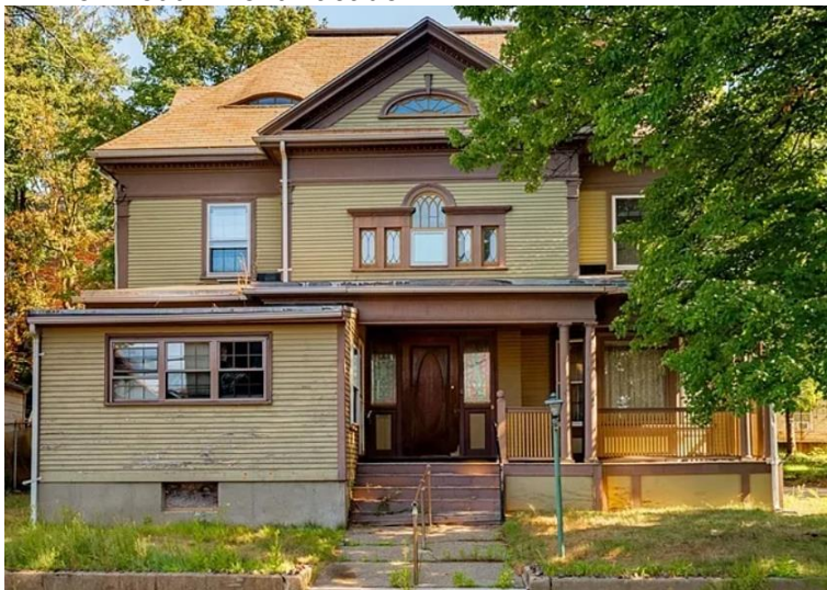
17 Monmouth Front Facade:
