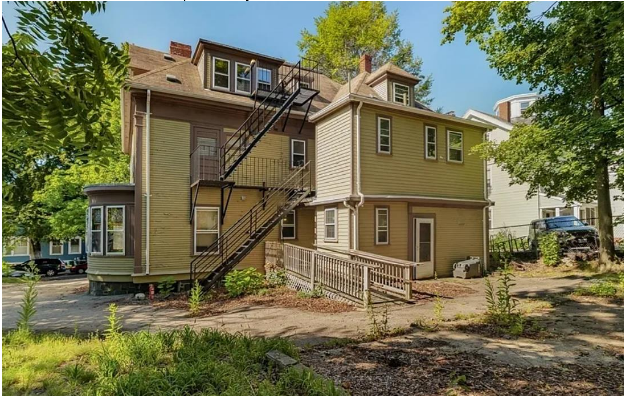
17 Monmouth Rear with Proposed Bay to be Demolished:
