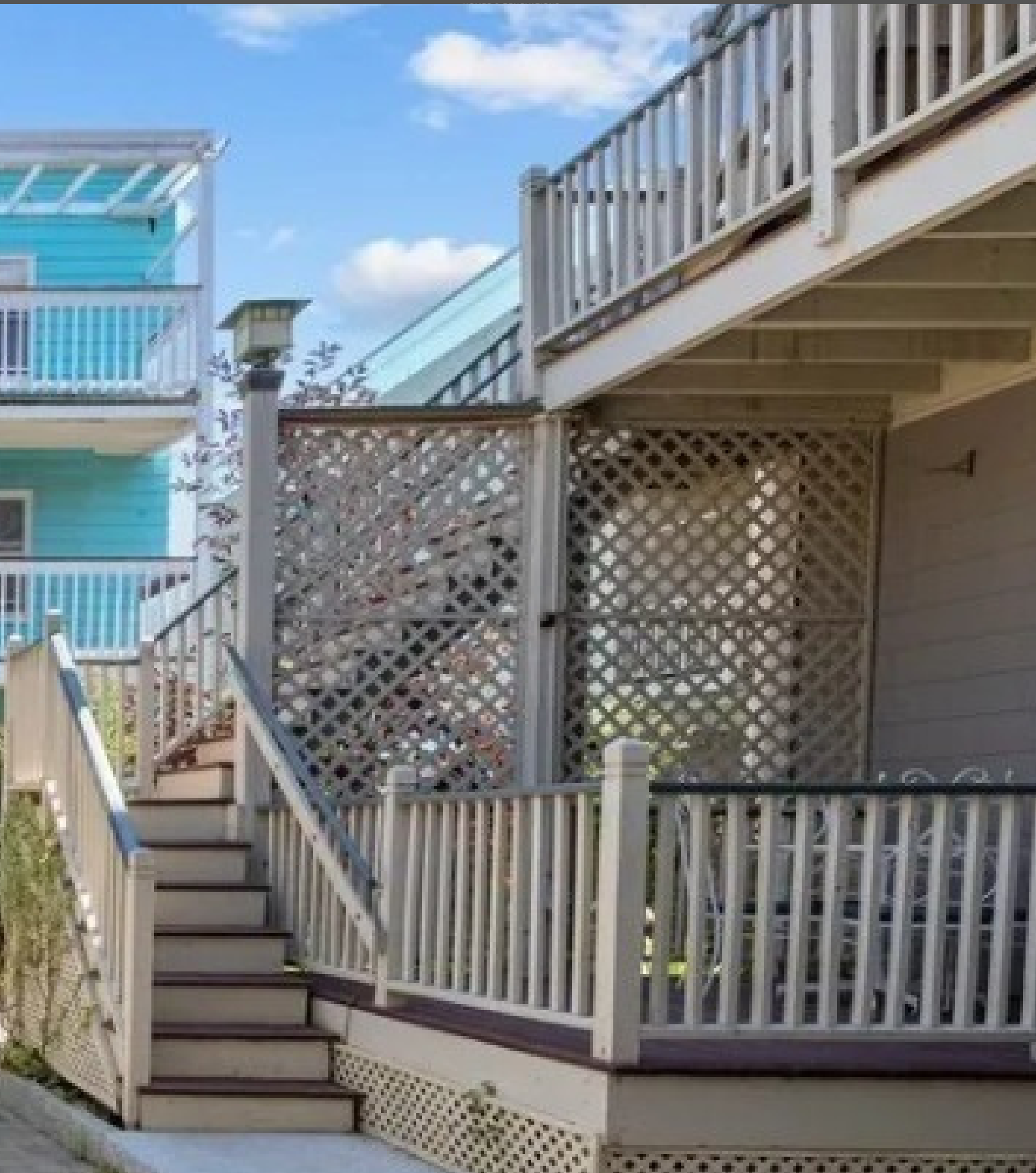
EXISTING LOWER DECK, STAIRS, RAILINGS AND LATTICE
