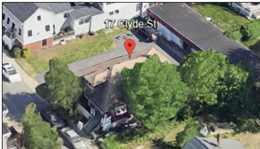
Google Imaging of 17 Clyde Street
