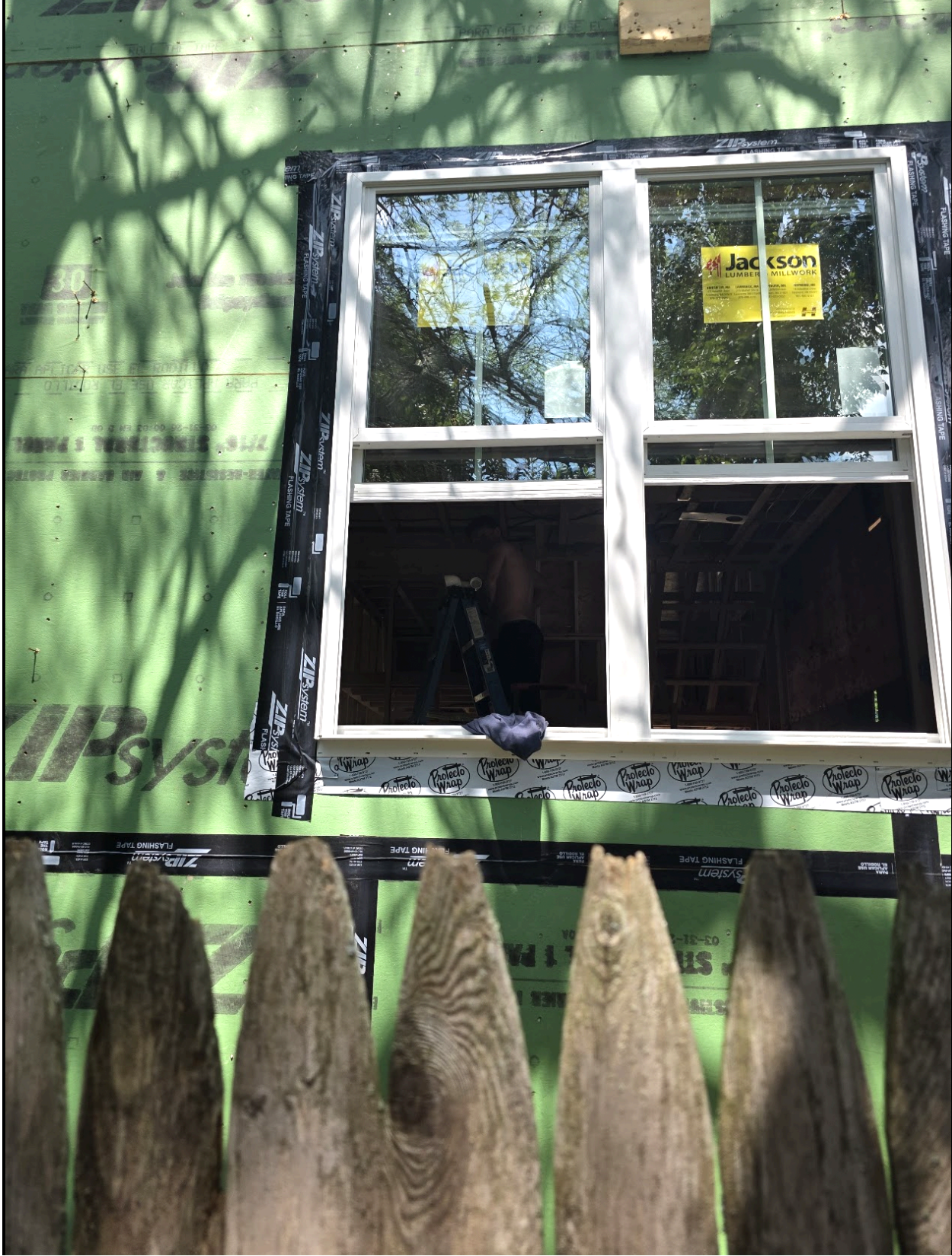
May 20 1:20pm. Worker on a ladder inside under-construction backyard cottage.
