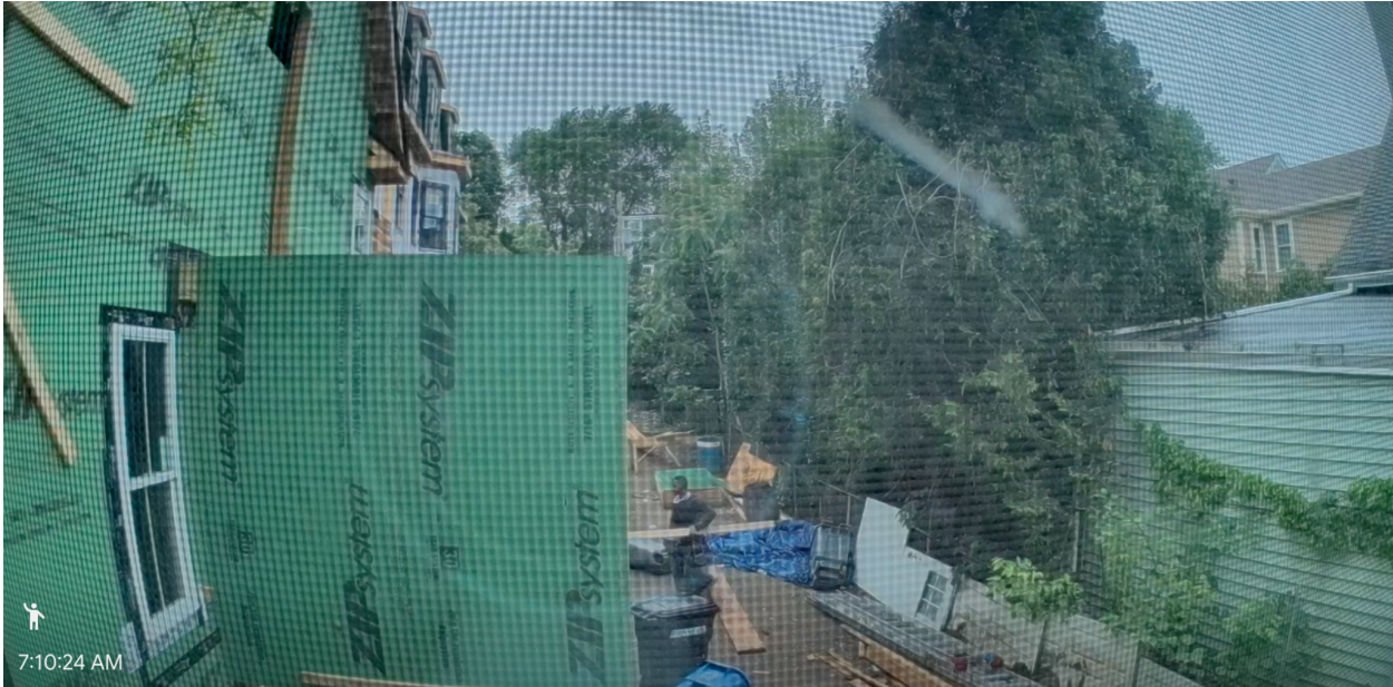
June 1: 7:10am worker entering the cottage construction site
