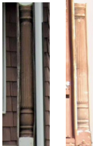
Above: 2 photos of the Tuscan column on right side of front porch
