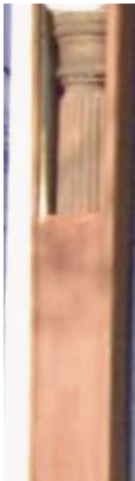
Above: Tuscan column on left side of front porch
