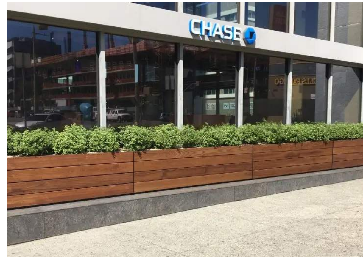
Lightweight Planters with Wood Cladding at Building Signage Canopy (Lv2)
