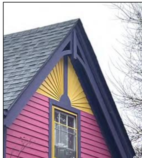
Existing Northern Elevation Pediment
