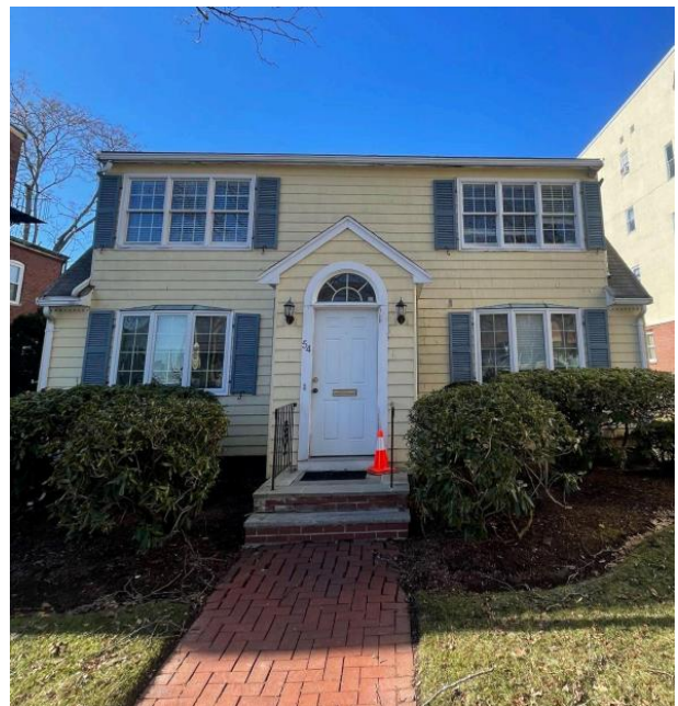
Front Elevation of 54 Highland Ave
