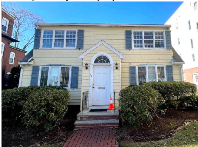
Front Elevation of 54 Highland Ave
