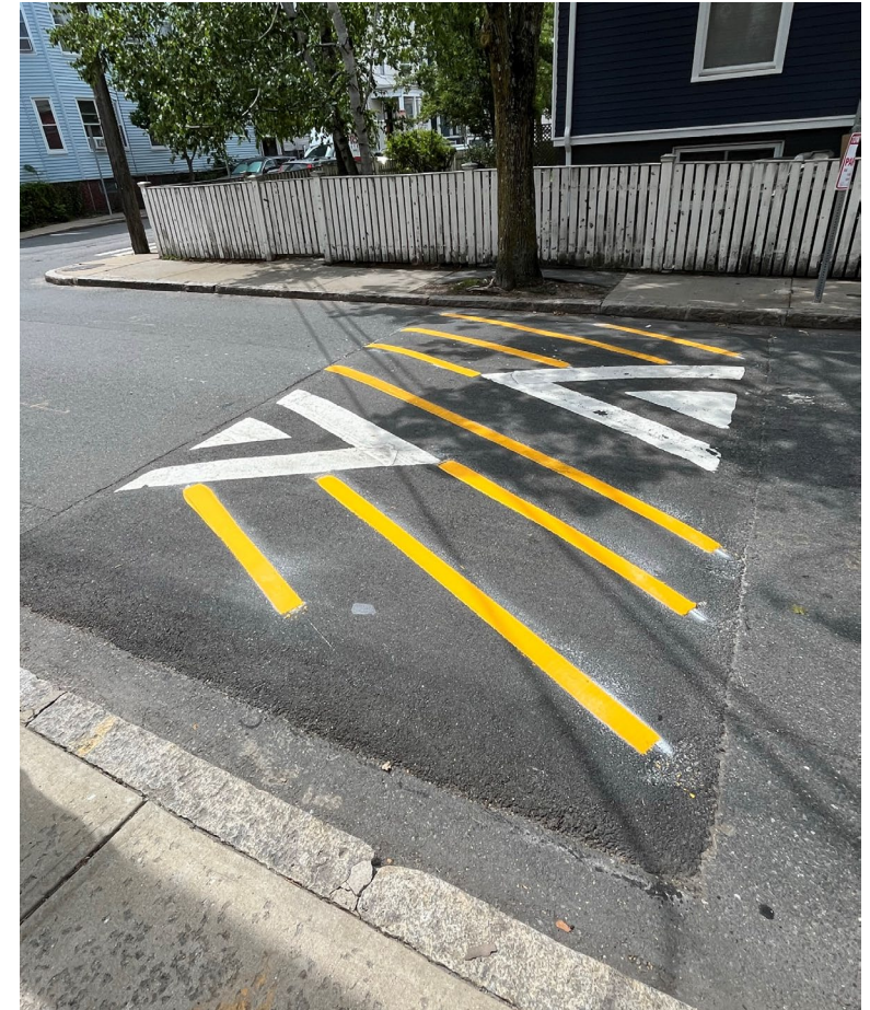
Freshly striped speed hump markings on Concord Ave at Dimick St
