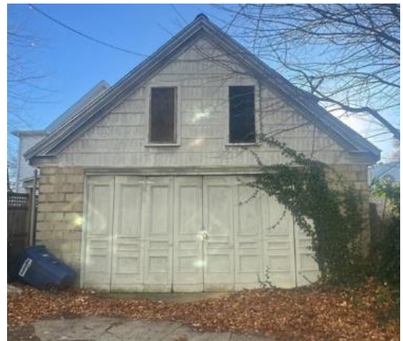
Front Elevation of the accessory structure at 141-143 Walnut St
