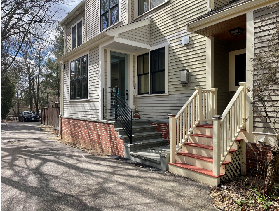
View from the driveway, showing the current rear parking
