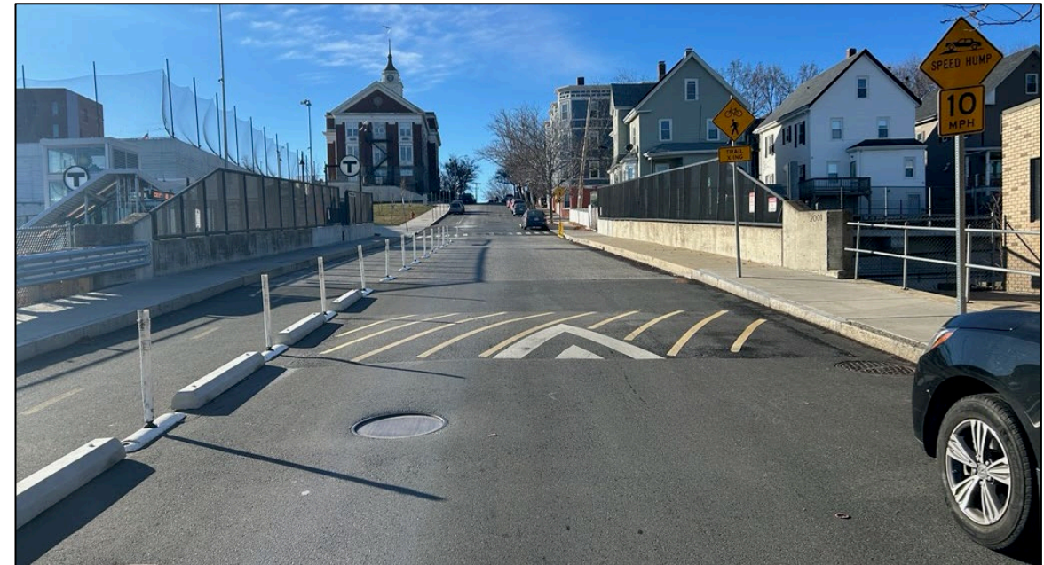
Pre-cast concrete curbs installed on School Street
