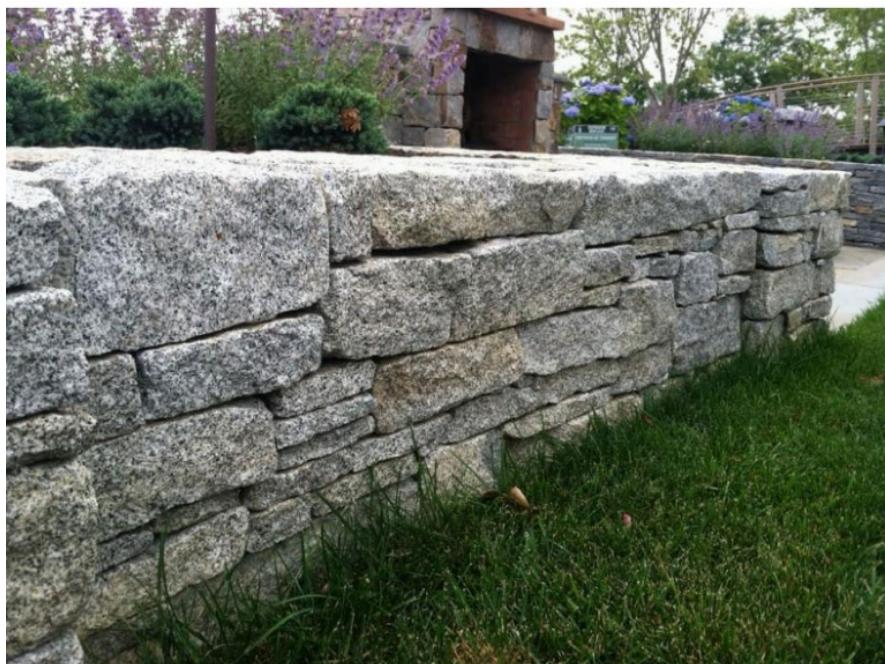
Above: an example of North Mountain Granite Wallstone, which is proposed for the retaining wall
