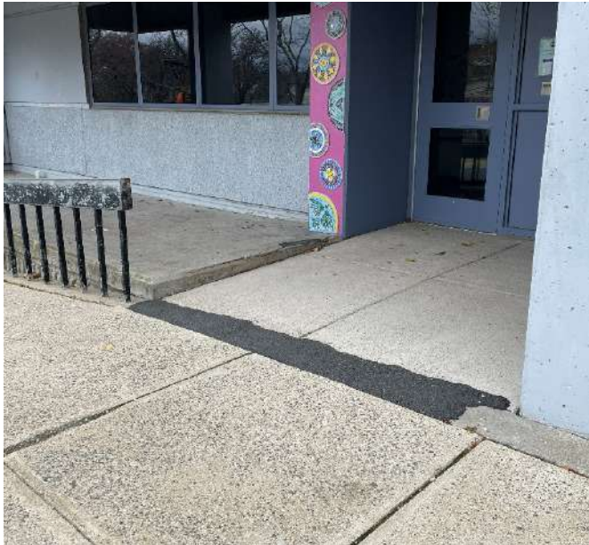
Non-accessible Ramps at North Entry
