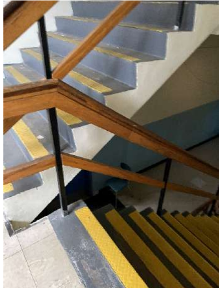
Open Guardrails
