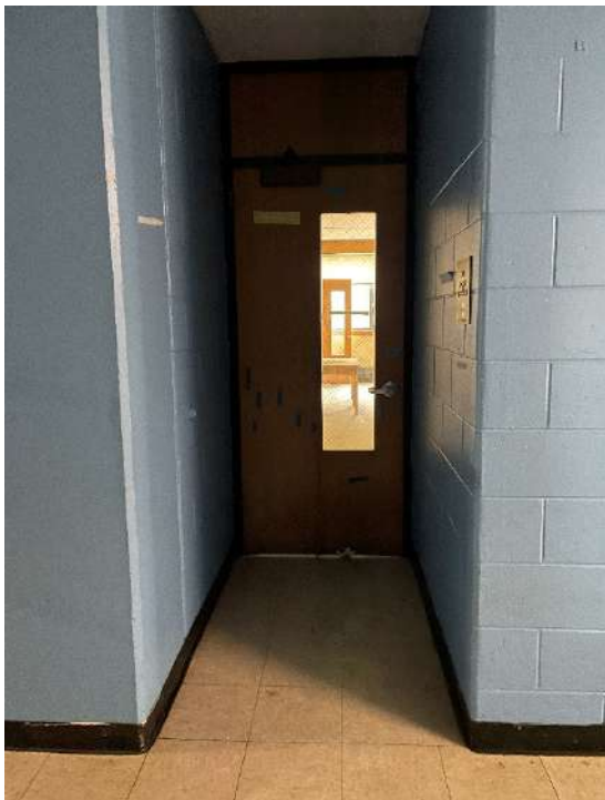
Non compliant Maneuvering Clearance
