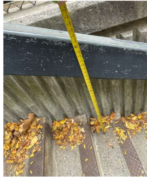
Non-compliant Handrails
