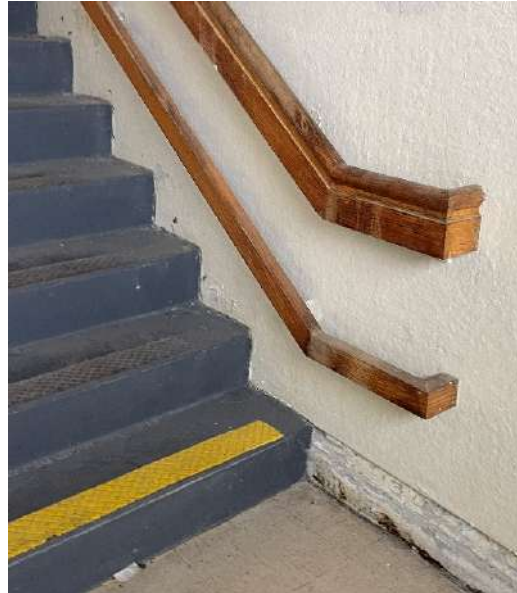
Non-compliant Handrails
