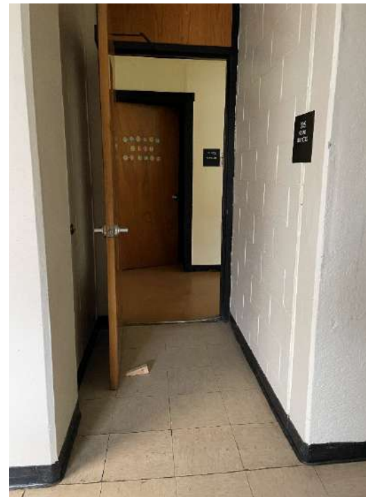
Non compliant Maneuvering Clearance
