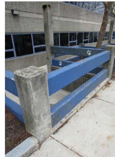
Low and Open Guardrails
