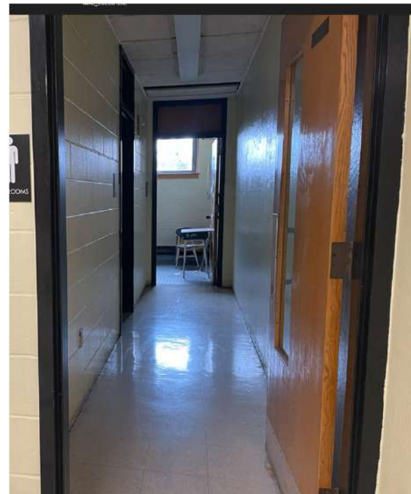
Non compliant Maneuvering Clearance
