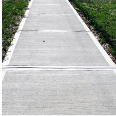
Cast-in-Place Concrete Paving
