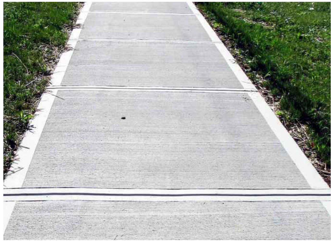
CAST-IN-PLACE CONCRETE PAVING
