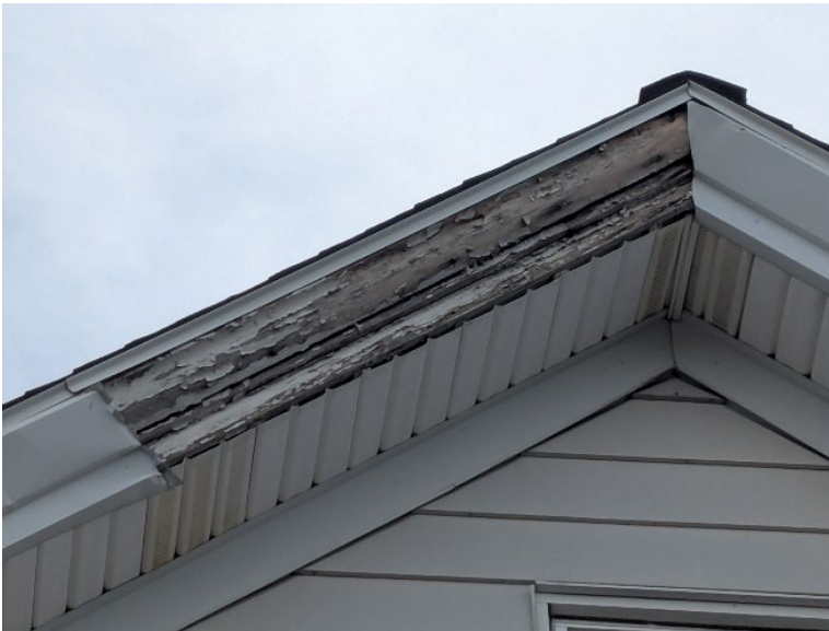
Photograph March 18, 2025, showing original eave rake trim under aluminum siding
