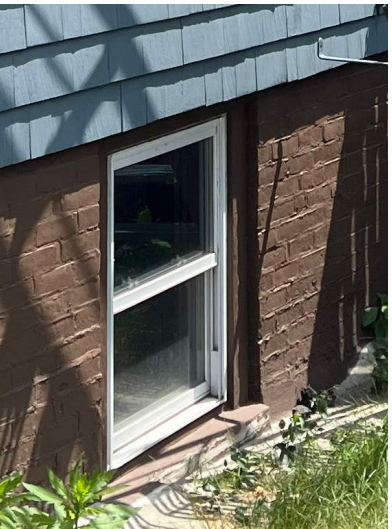
4 PAINTED BRICK MASONRY FOUNDATION WALLS
