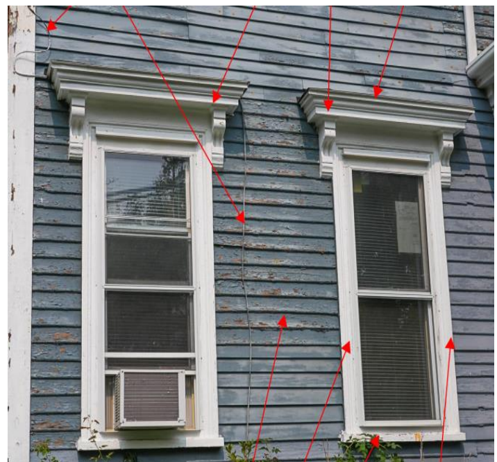
Above: Current photo of the front elevation identifying proposed changes to window header frieze board/crown and cap, window casings trimboards, window sills, and back-band.
