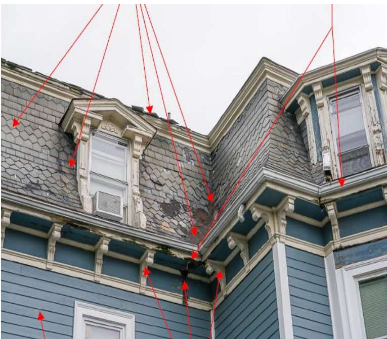
Above: Current photo of the second story and half-story of the left side elevation identifying brackets, soffits, and slate roofing.
