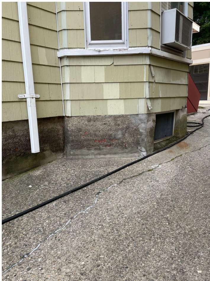
Fig. 9 - Detail of foundation parging
