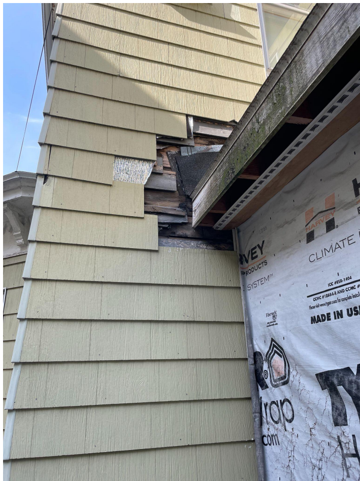
Fig. 7 - Detail of siding below asbestos
