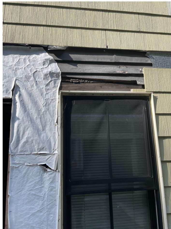
Fig. 8 - Detail of siding below asbestos
