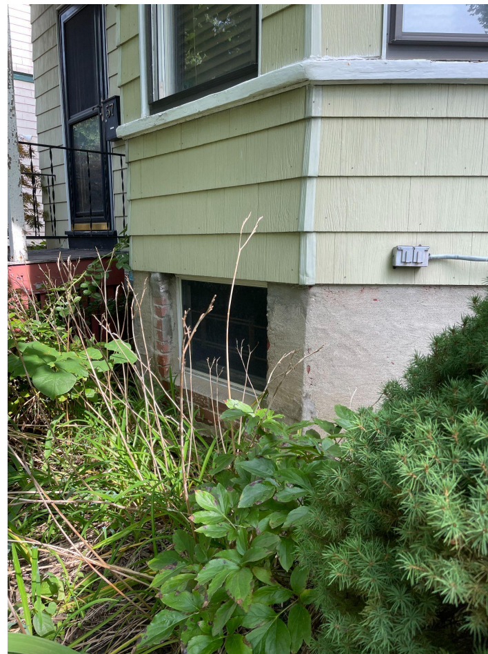
Fig. 10 - Detail of foundation parging
