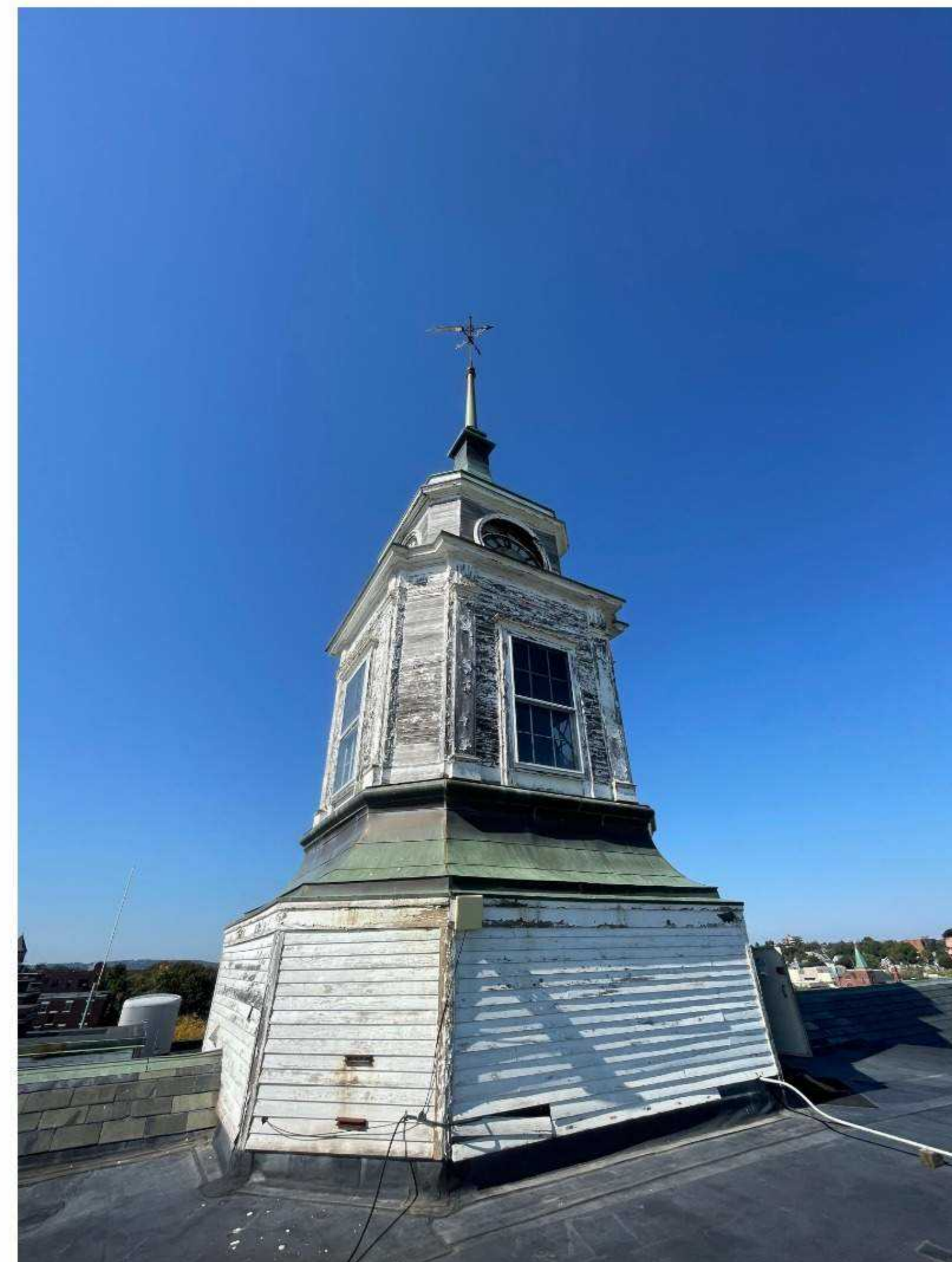
Cupola and surrounding Roof(s)
