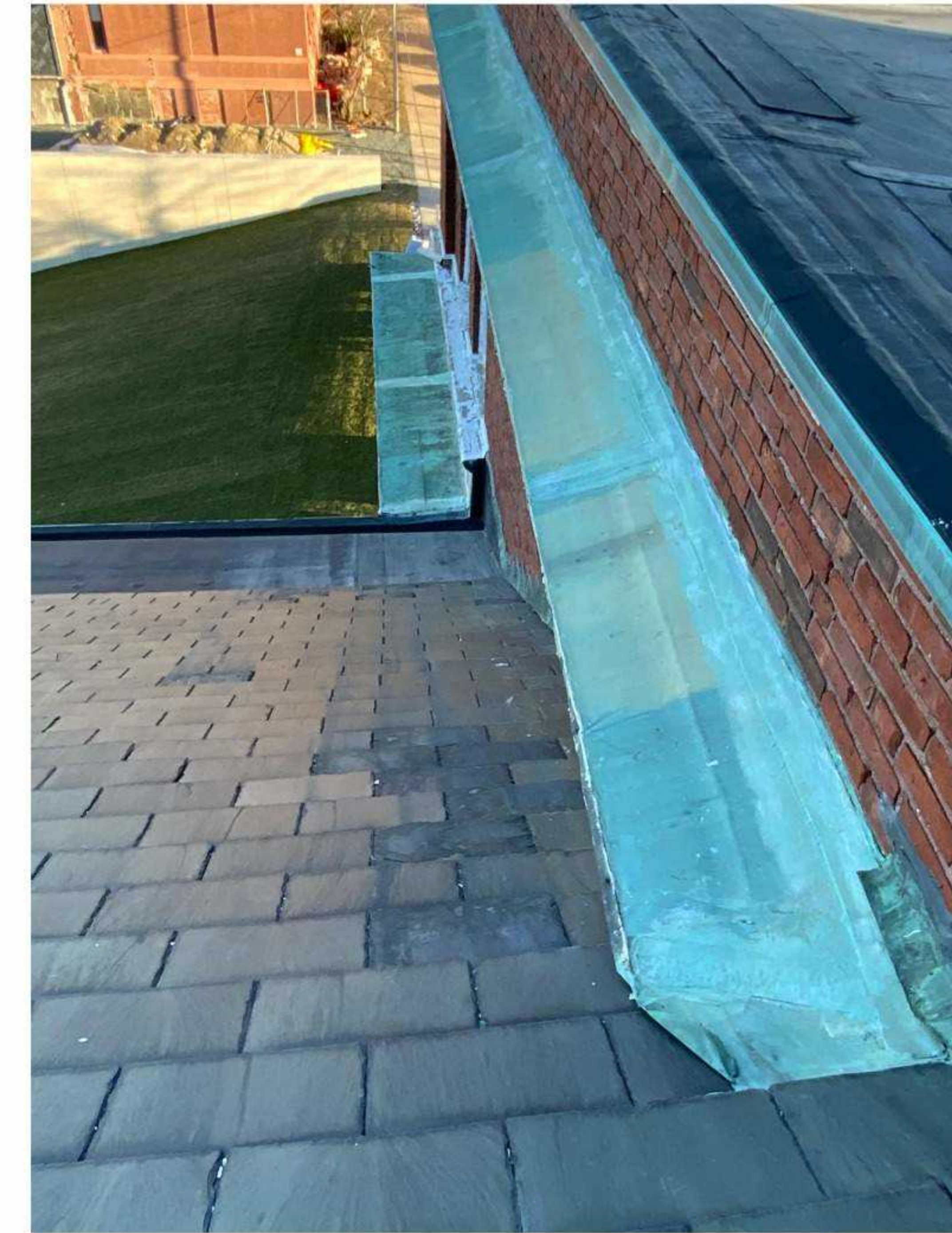
Existing Slate Roof and Brick
