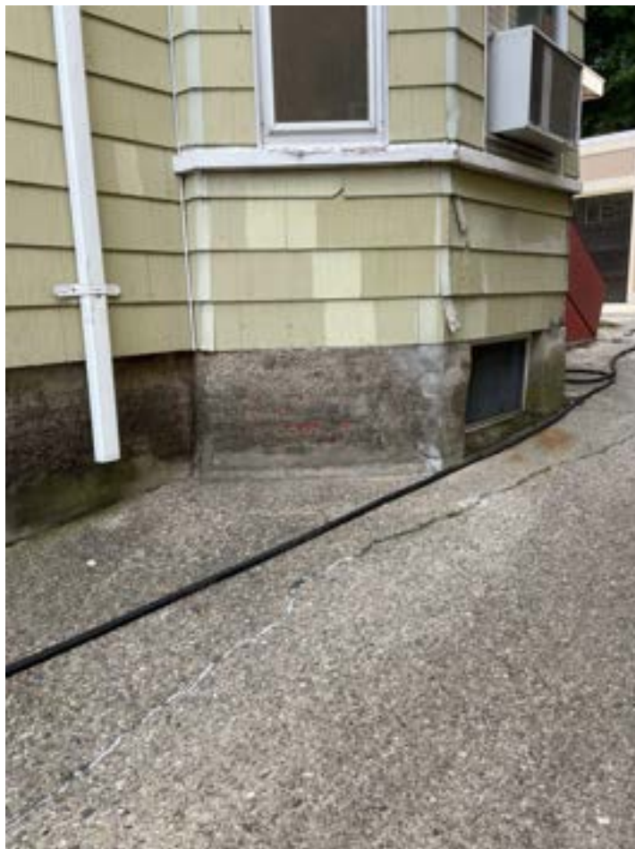
Fig. 9 - Detail of foundation parging
