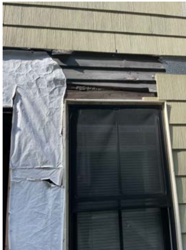
Fig. 8 - Detail of siding below asbestos
