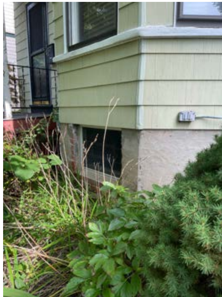
Fig. 10 - Detail of foundation parging
