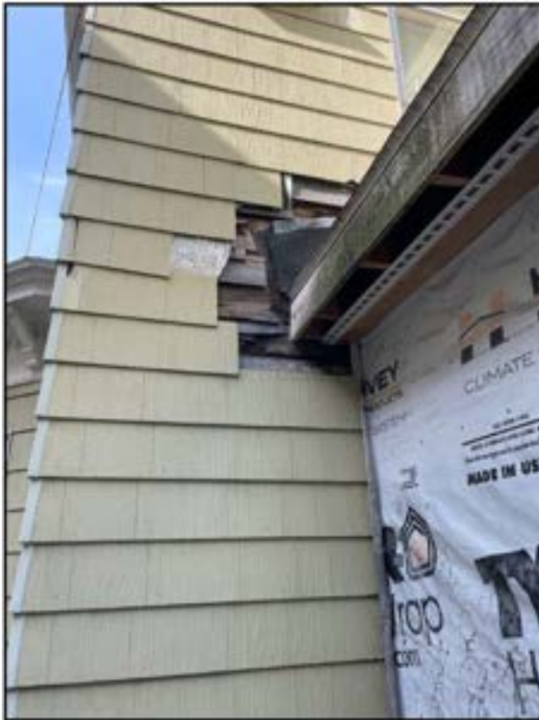
Above: Detail of exposed wood clapboard below asbestos clapboard
