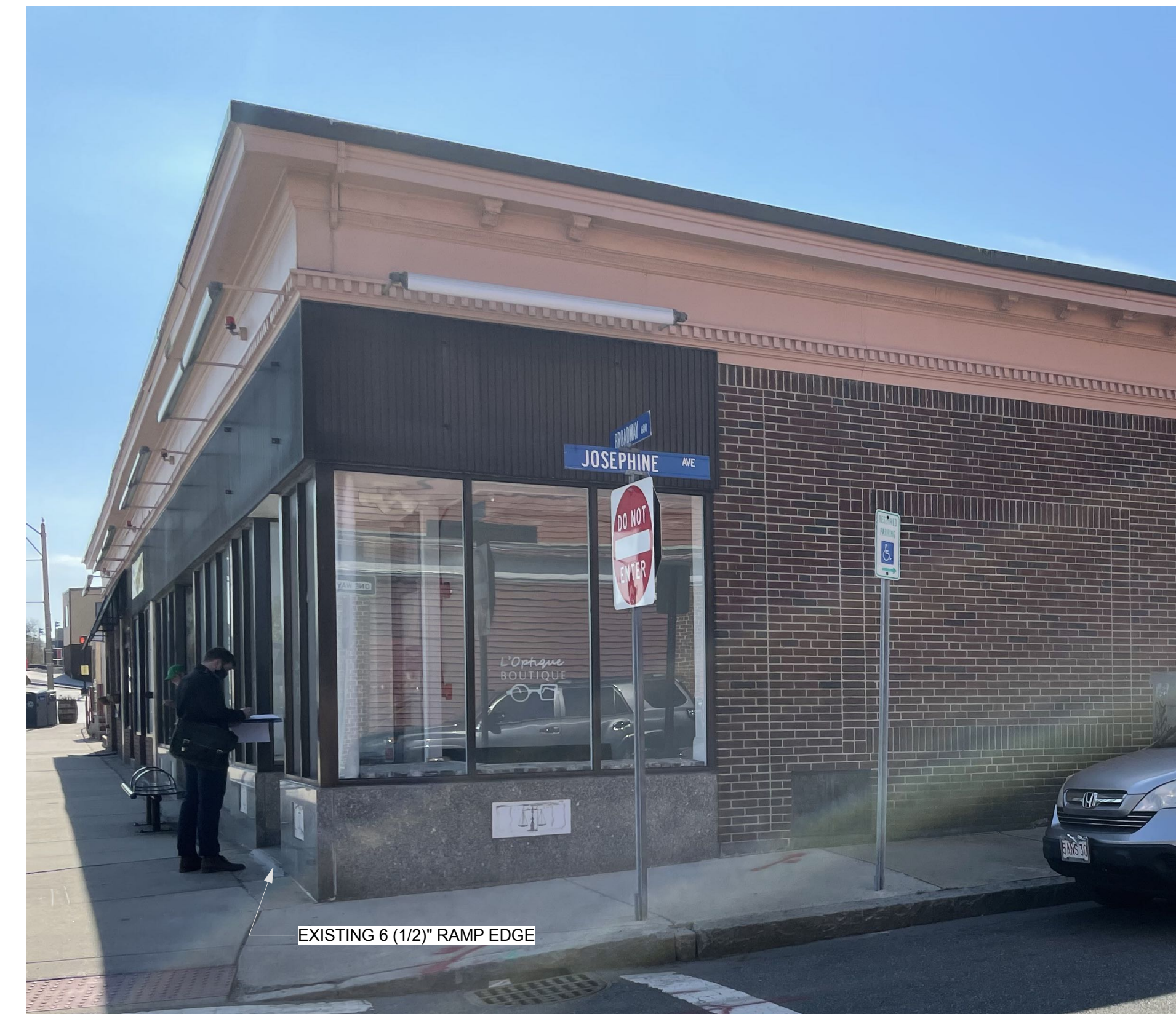
2 VIEW OF PROJECT SITE FROM ACROSS JOSEPHINE AVENUE
