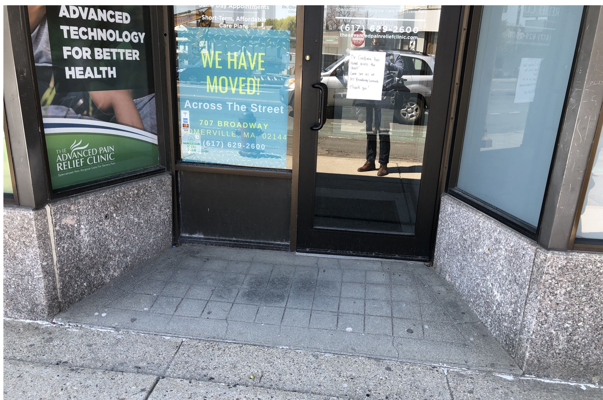
3 EXISTING ENTRY RAMP, EXTERIOR
