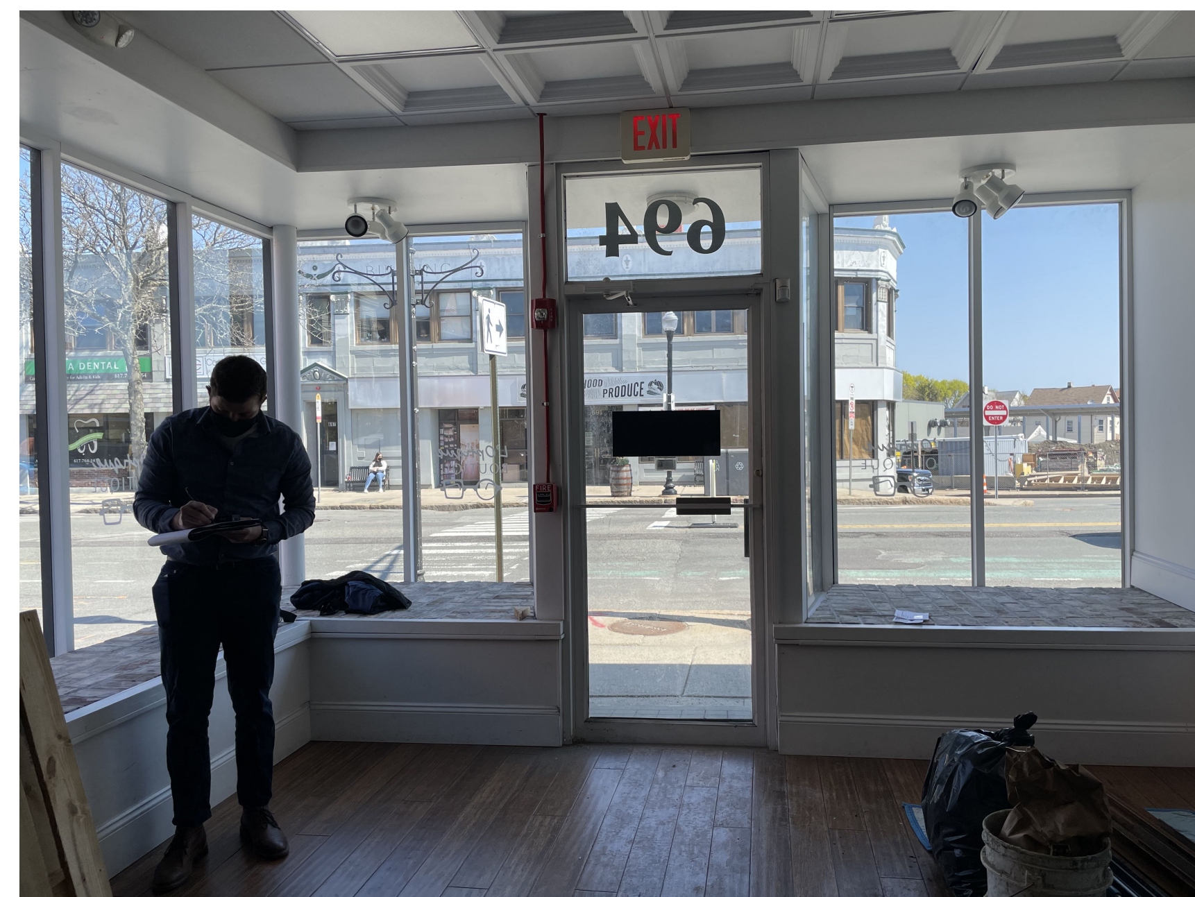
4 EXISTING ENTRY, INTERIOR
