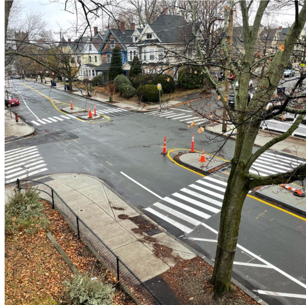
New pedestrian refuge islands and temporary pavement markings on College Avenue
