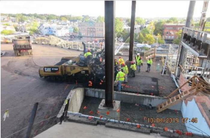
October 2019: Workers Prepping the Paver for Paving the Temp Access Road PH 1
