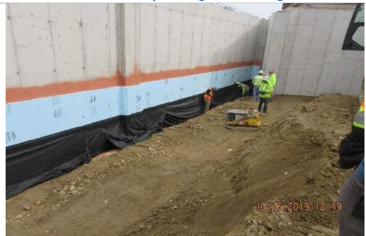
October 2019: Backfilling and Compacting Foundation Wall After Waterproofing & Insulating PH 2
