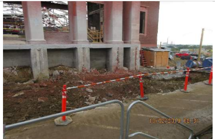
October 2019: Backfilling and Compacting Foundation Wall After Waterproofing & Insulating PH 2
