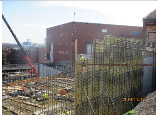
April 2019: Lower Level Foundation Wall Rebar (Next to 1895 Building)
