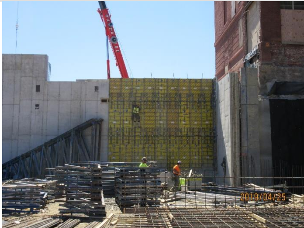
April 2019: Lower Level Foundation Wall (One Sided Forms/Bracing)
