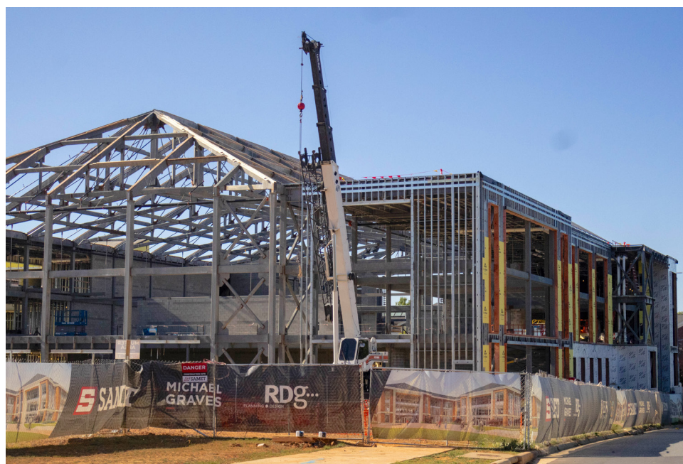
Slattery Center construction on May 3.
