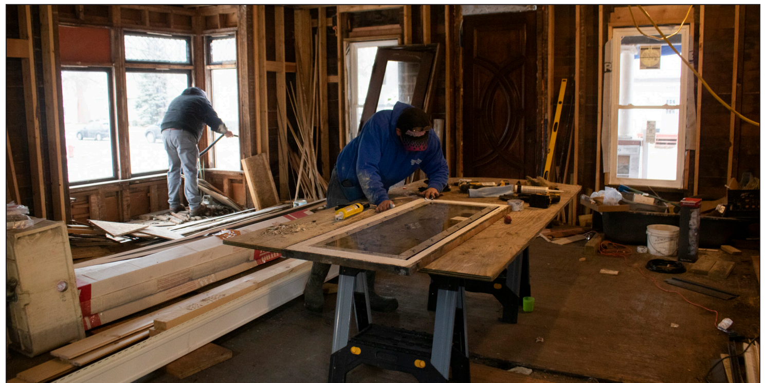
Contractors install new windows in Ken Williams house on Feb. 21, 2022.
