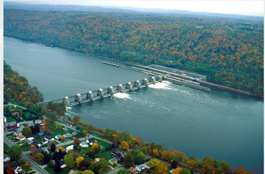
Aerial view from downstream side
