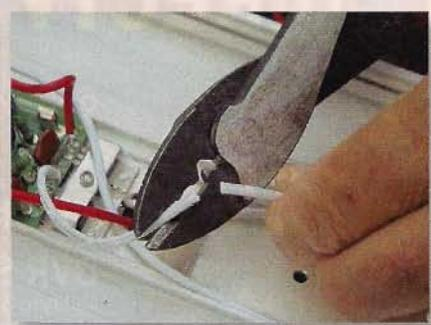
2) We cut the ground wire from the ballast to the switch.
