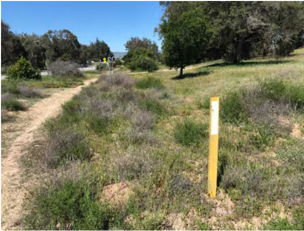
Photograph 7. View of a gas pipeline marker located along the southern boundary of the subject property, facing west.
