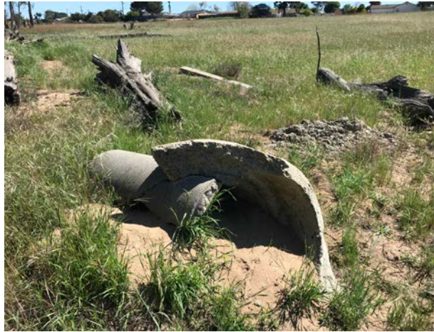
Photograph 8. View of concrete debris located in the southwestern corner of the subject property, facing northeast.
