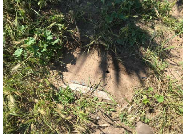
Photograph 3. View of a water meter located along the eastern boundary of the subject property.
