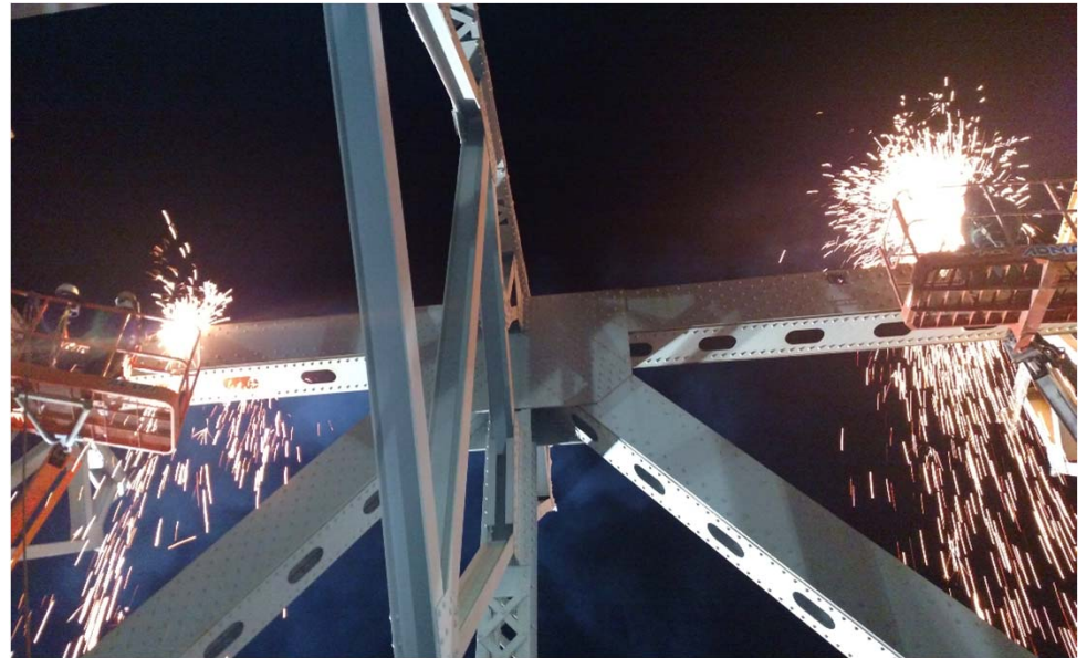
Torch cutting former Tappan Zee Bridge - Albany, New York
