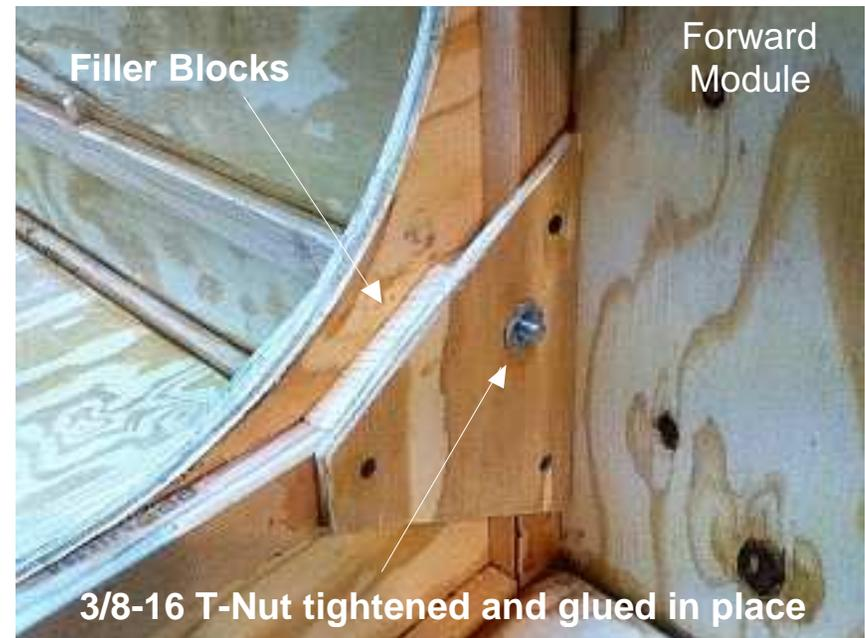
Quick-Set Epoxy is recommended to secure the T-NUT.
