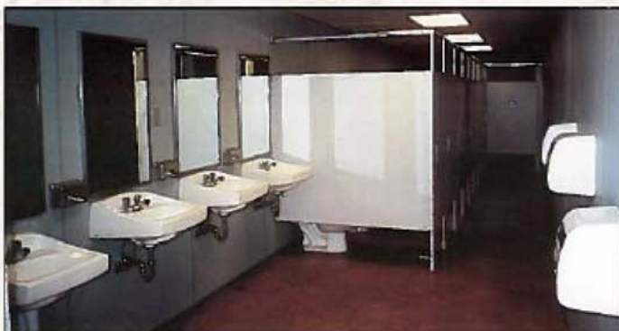
New restrooms beneath the south grandstand will be used for the JUCO Tournament for the first time: $130,000 – Alpine JUCO & PIAB Project.
