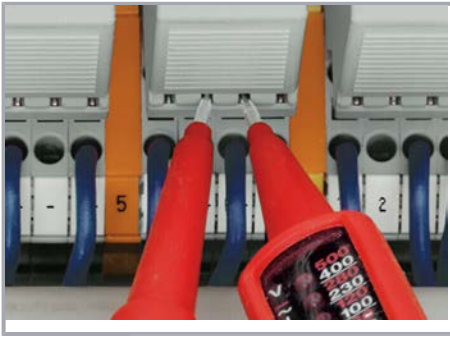
Function testing via touch-proof test slots
