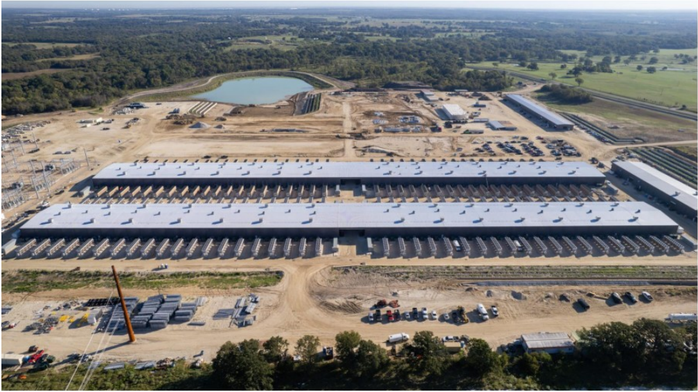
400 MW Phase I at Corsicana Facility - Corsicana, Texas
