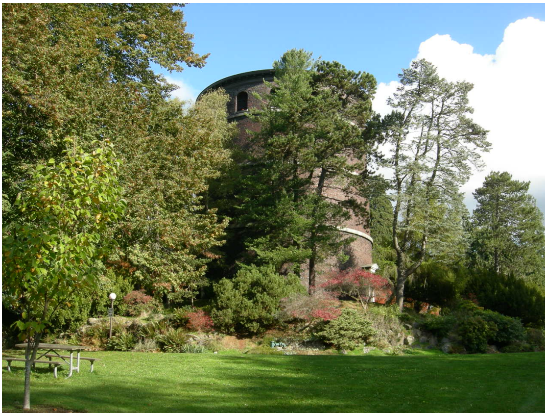
Photo 14 – Water Tower, west side, October 2010
