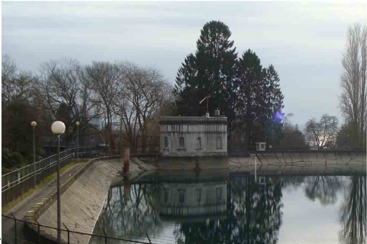
Photo 10 – Gate House, northeast side, February 2009
