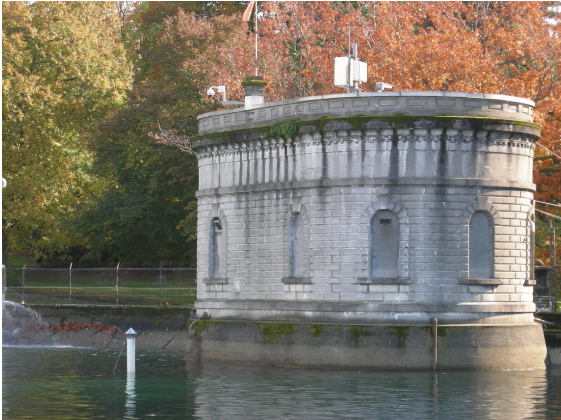
Photo 9 – Gate House, north side, October 2010
