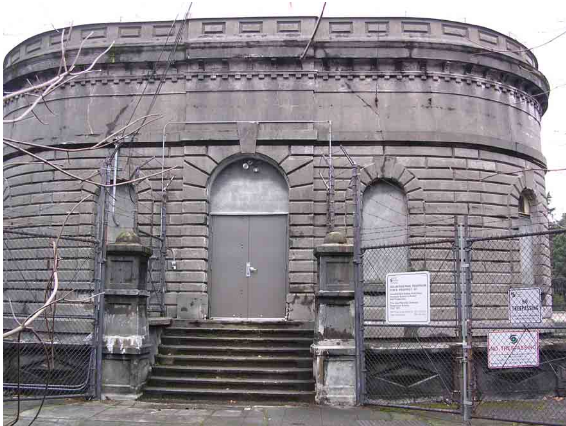
Photo 7 – Gate House, south side, January 2007
