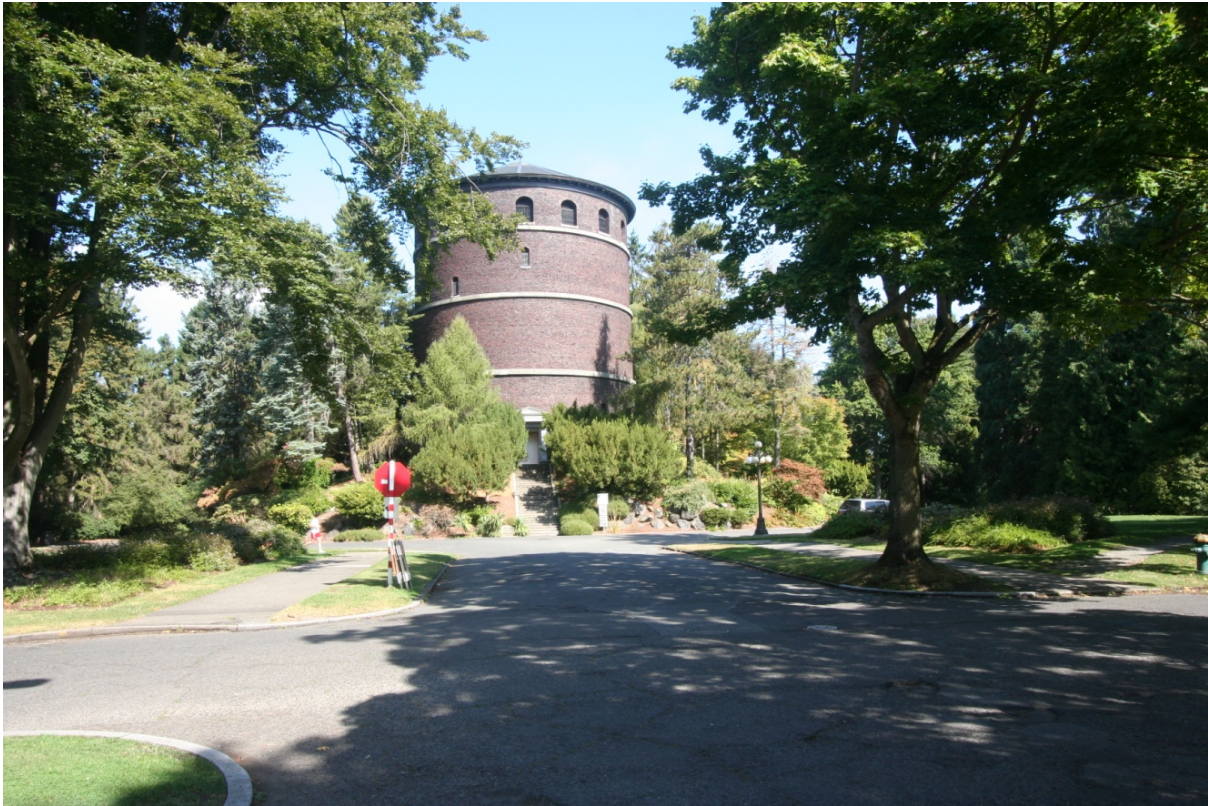
Photo 11 – Water Tower, south side, September 2006
