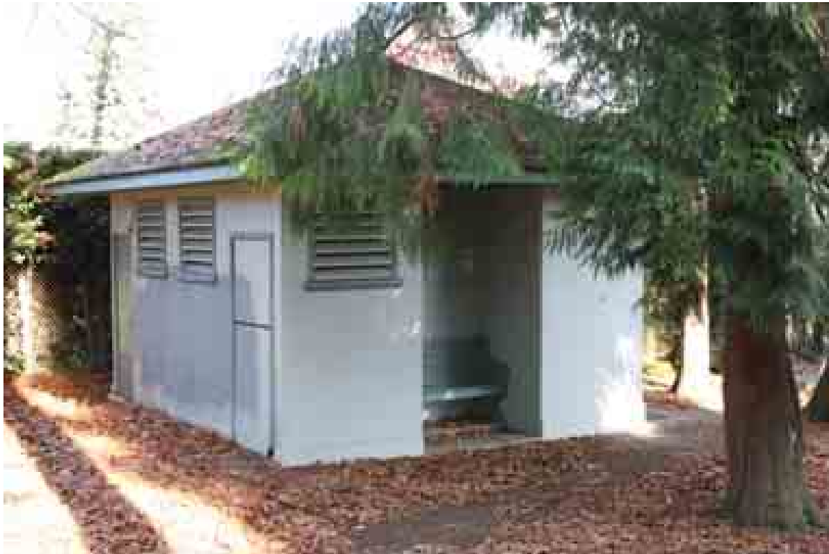
Photo 19 – Comfort Station, south and west sides, February 2008
