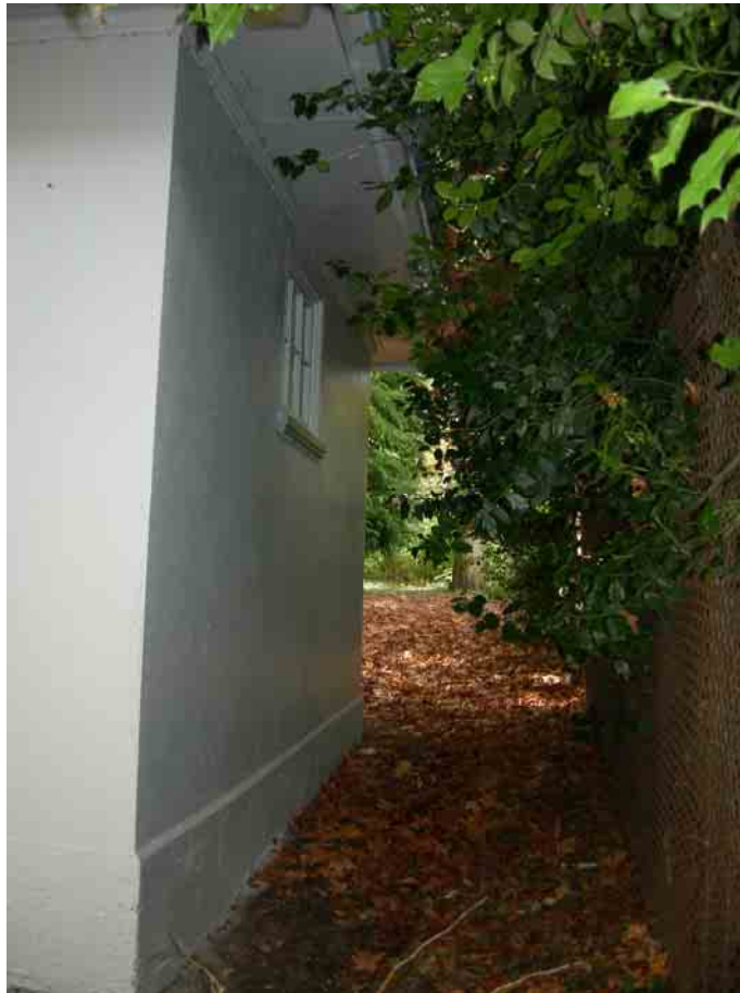
Photo 21 – Comfort Station, north side, October 2010
