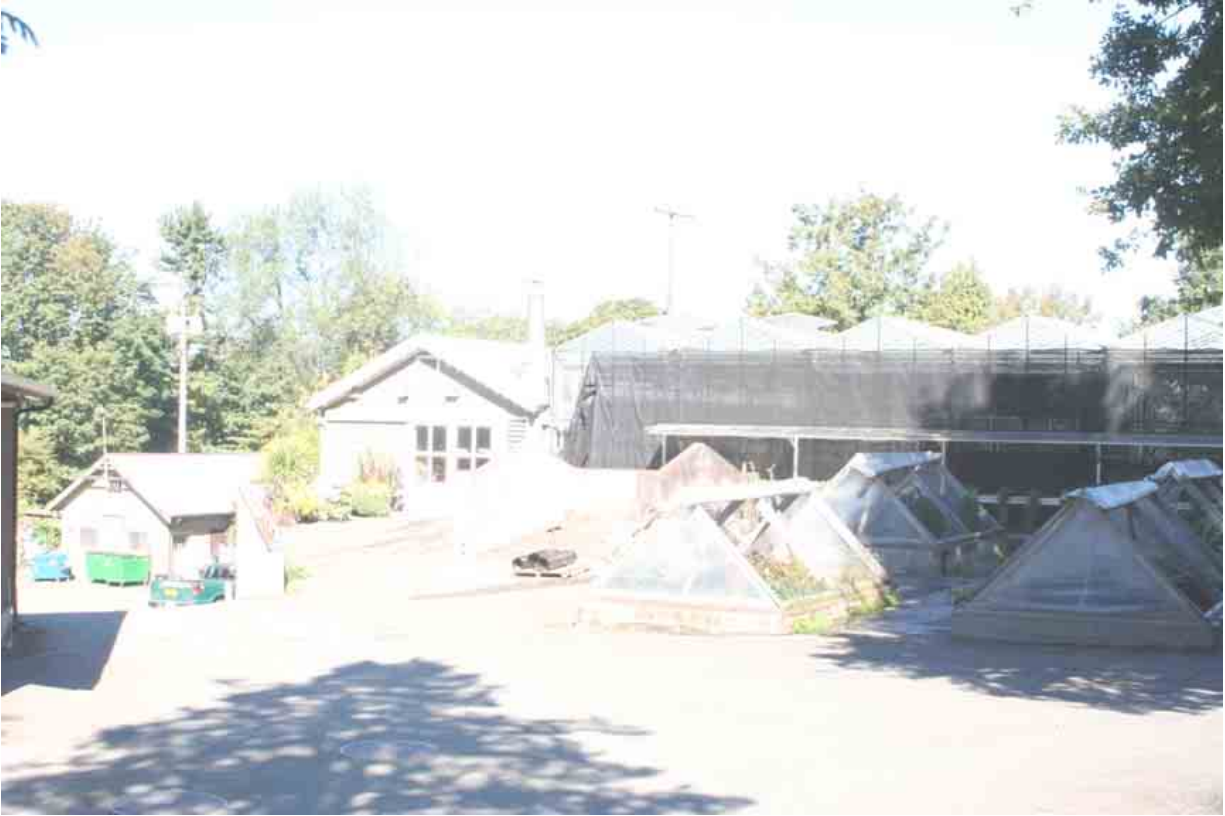
Photo 23 – Maintenance Facilities, south side, September 2007
