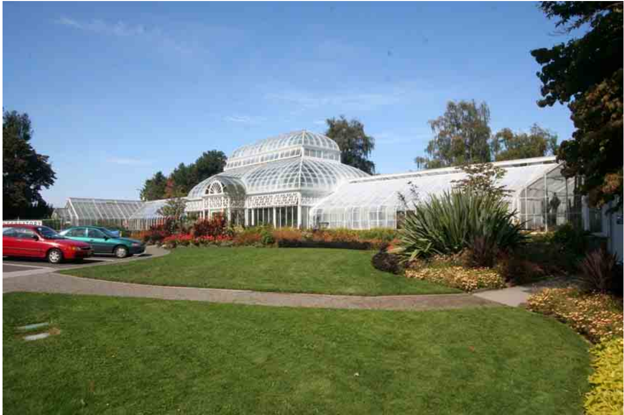
Photo 25 – Conservatory, south side, September 2009
