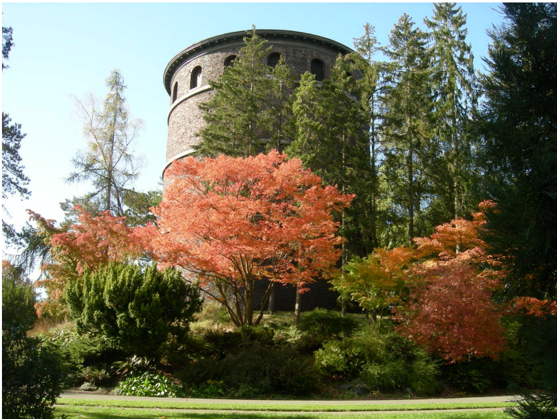
Photo 13 – Water Tower, east side, October 2010
