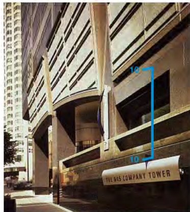
BASE OF BUILDING AT ENTRANCE
