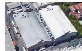
WARNER BROS. INFILL BLDGs. PROTOTYPE BUILDING BETWEEN STAGES (22' X 300') Burbank, California Completed: 2008, 2010 Size: 13,000 SF & 9,500 SF Role: Technical Lead Architect: HLW
