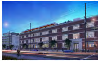
COCA COLA BUILDING WAREHOUSE TO CREATIVE OFFICE CONVERSION Los Angeles, California Projected Completion: 2017 Size: 110,000 SF Role: Technical Lead Architect: HLW
