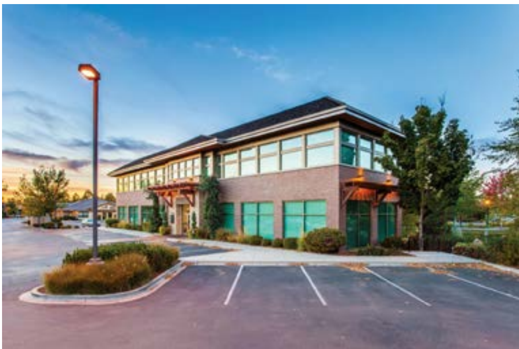
Image 3: Ample space to back out, low shrubbery to not obstruct sightlines, accessible parking connects to sidewalk.
